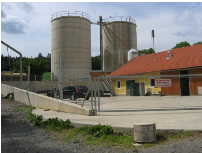
Photograph 6.2: Standing silos for corn and cover of underground main digester 1.
